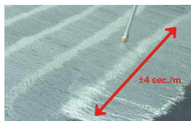
Spray time is ± 4 seconds per m.
